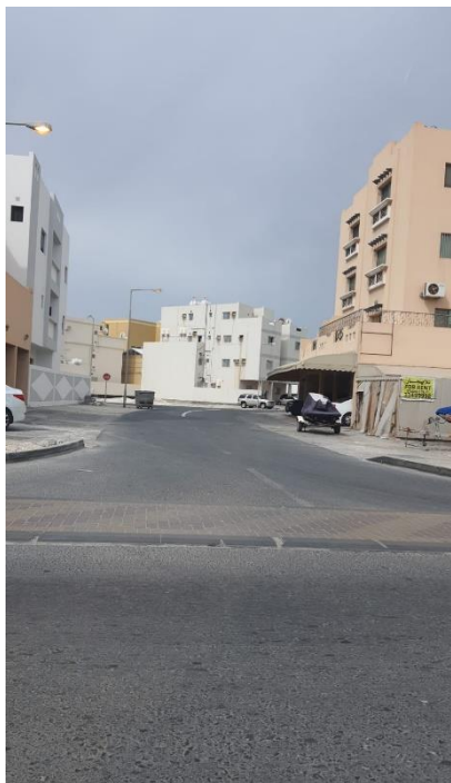
Figure 4.15: New Hidd Lack of sidewalks (Akram)
