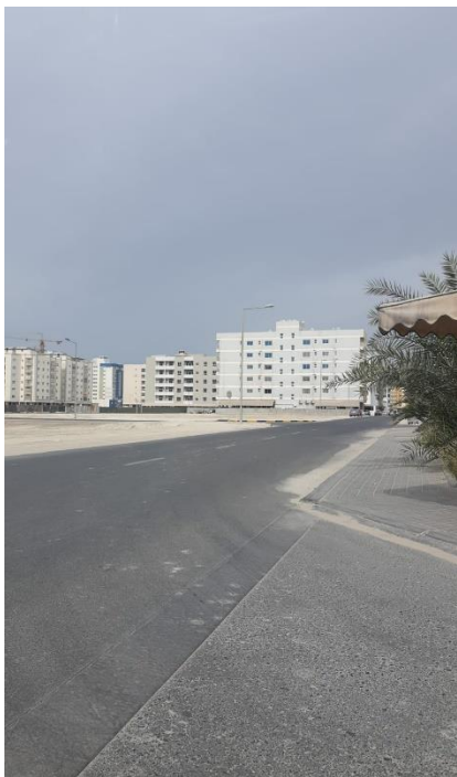
Figure 4.14: New Hidd empty plots and lack of walkway (Akram)
