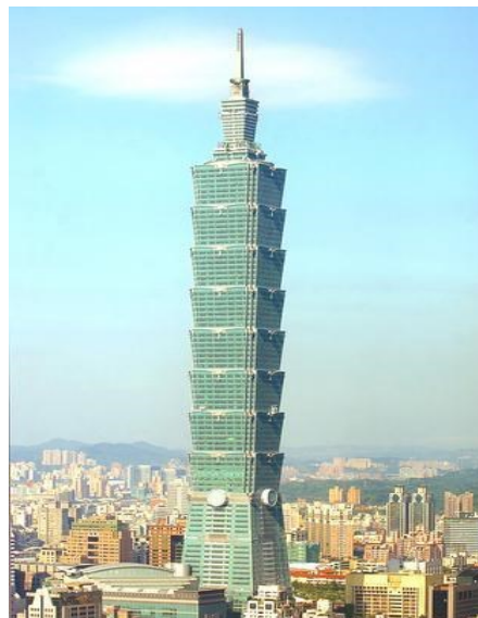
Figure 2.9 Taipei101 in Taiwan (source: WIKIARQUITECTURA, 2021)
