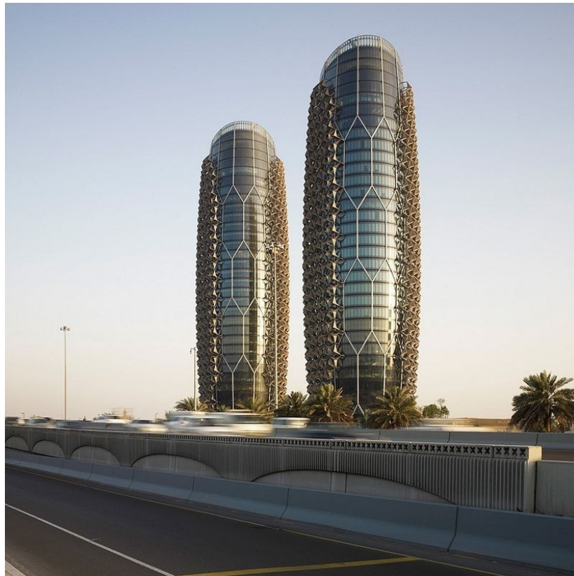
Figure 5.9 The Al Bahar Towers in Abu Dhabi (source: Albayan, 2015)
