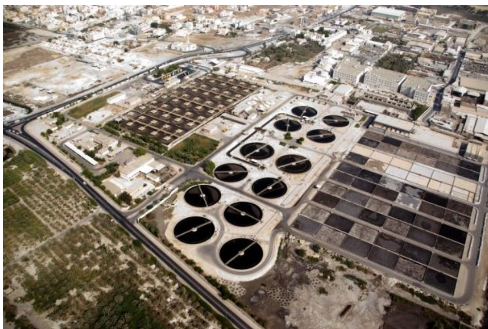
Figure (4-25) Tubli Sewage Treatment Plant (STP)
