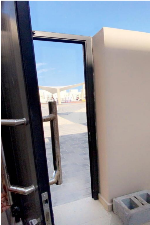
Fig. 4.17: The New External Door Facing the Exterior Garden
