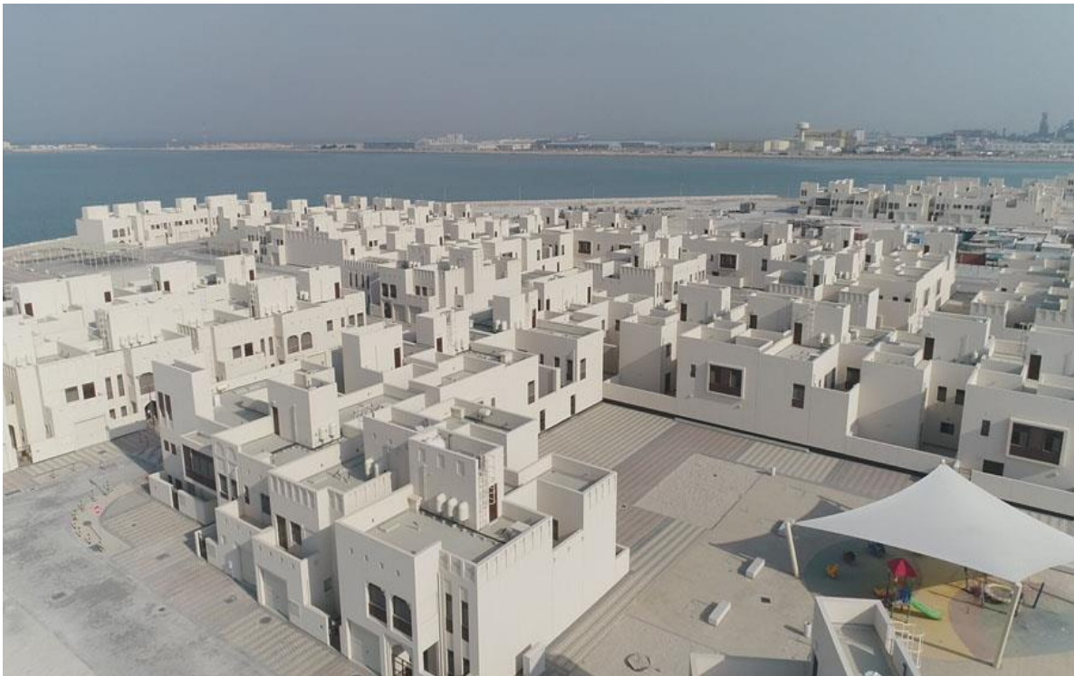
Fig. 3.1: East Hidd Housing Project (Source: Project Management International Systems - PMIS, 2023)
