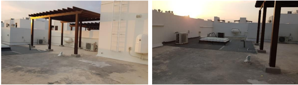
Figure (10): Main restriction affecting PV application.
