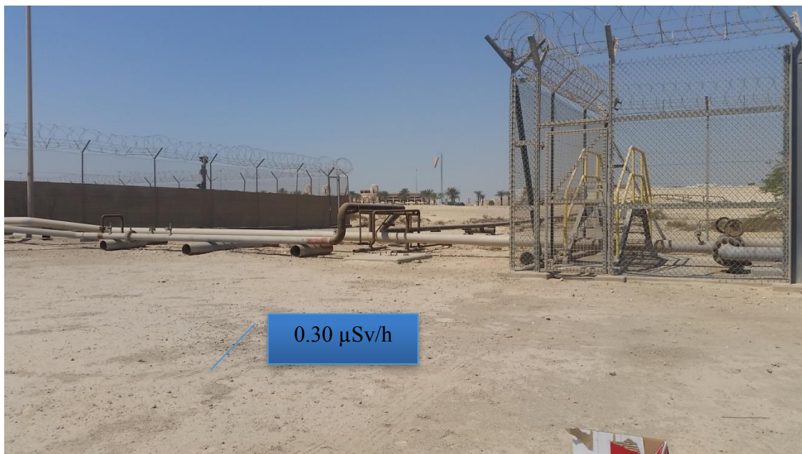
Figure (10) Pipelines installations on 96 Highway
