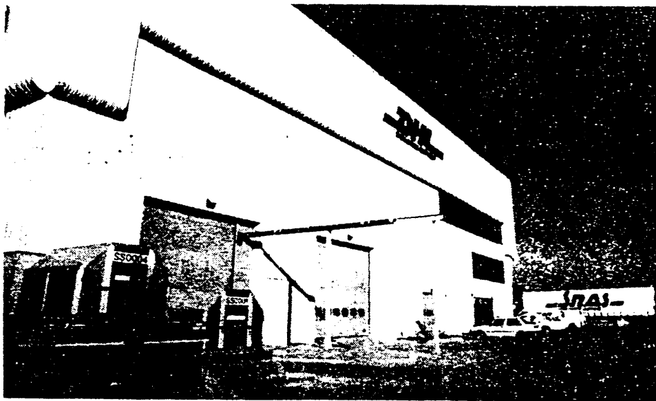
●The DHL Regional Distribution Centre at Bahrain International Airport.
