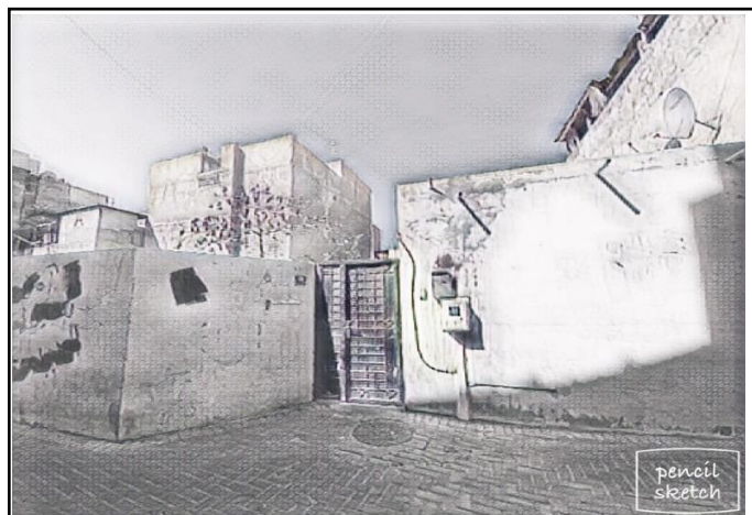
Fig 4.1 Courtyard house façade (Source:Author)
