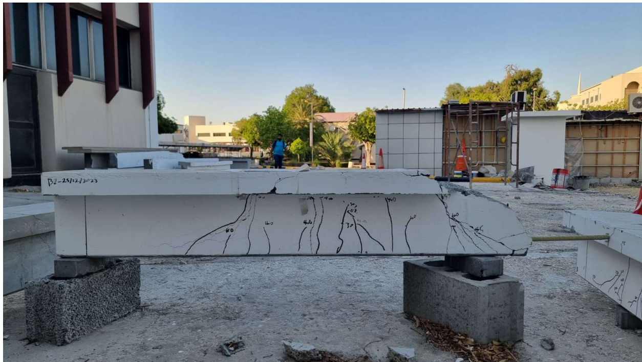
Figure A2. 2: Crack pattern of beam GT-2.7-50-16
