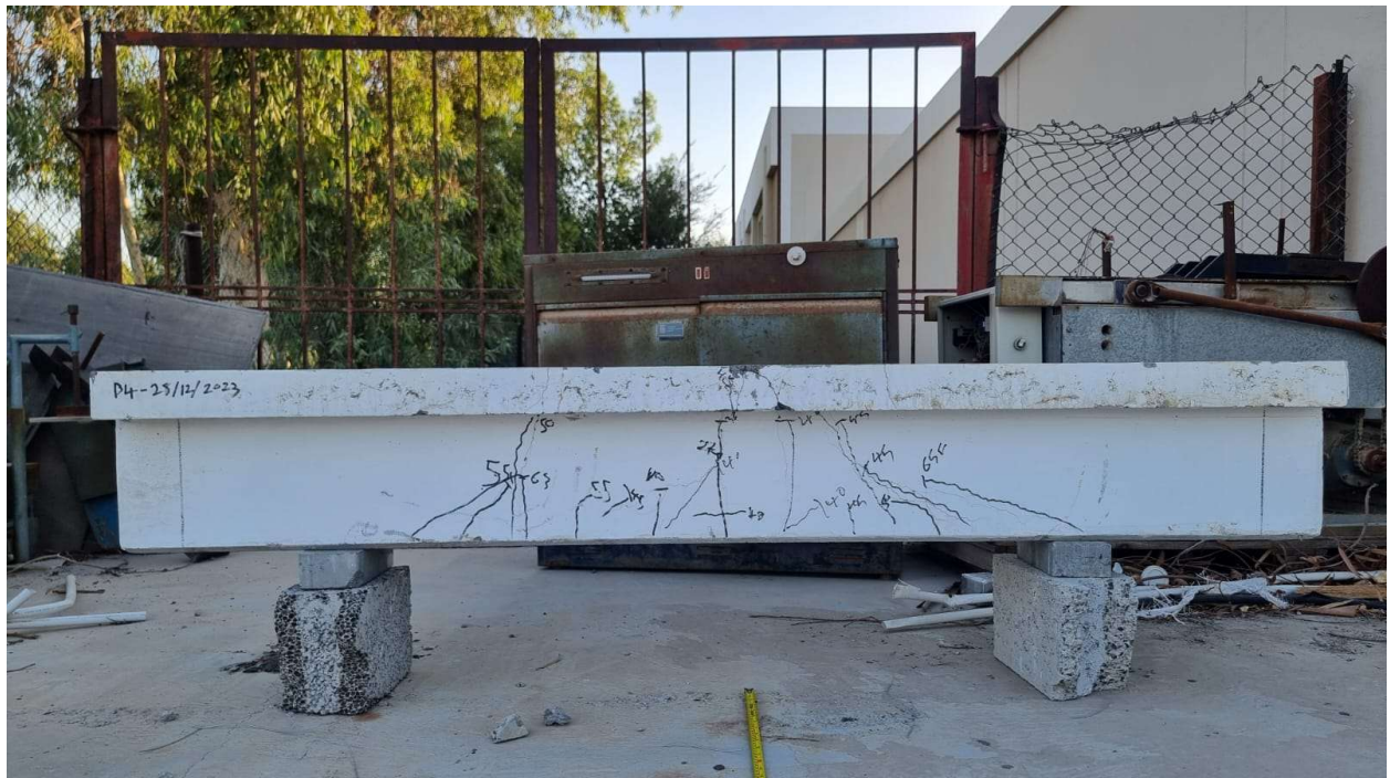
Figure A2. 2: Crack pattern of beam GT-3.5-60-16
