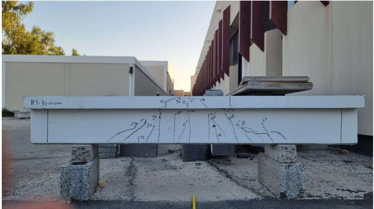
Figure A2. 3: Crack pattern of beam GT-3.5-40-16
