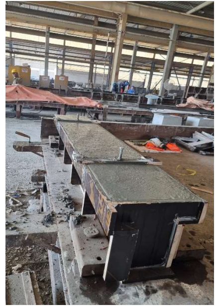
Figure 3.6: Beams Concreting process: (a) concrete batching, (b) concrete pouring using a bucket, (c) surface leveling and vibration, (d) completed beam after casting
