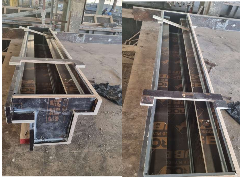
Figure 3.3: T-beam formwork
