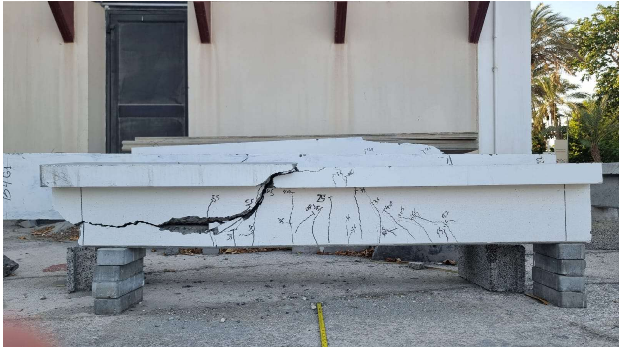
Figure A2. 1: Crack pattern of beam GT-3.5-50-16
