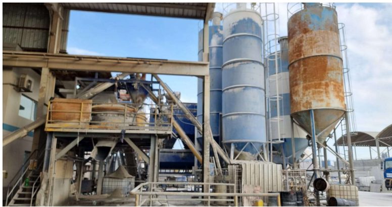
Figure 3.5: Automatic concrete mixer used for concrete mixing
