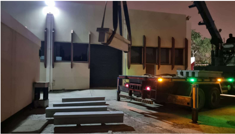
Figure 3.8: Beams Transportation
