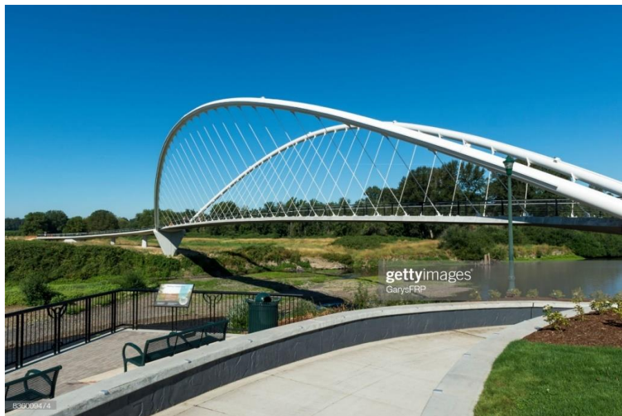
Figure 1-5 Riverfront Park Minto Island Bridge in Salem Oregon (gettyimages, n.d.)
