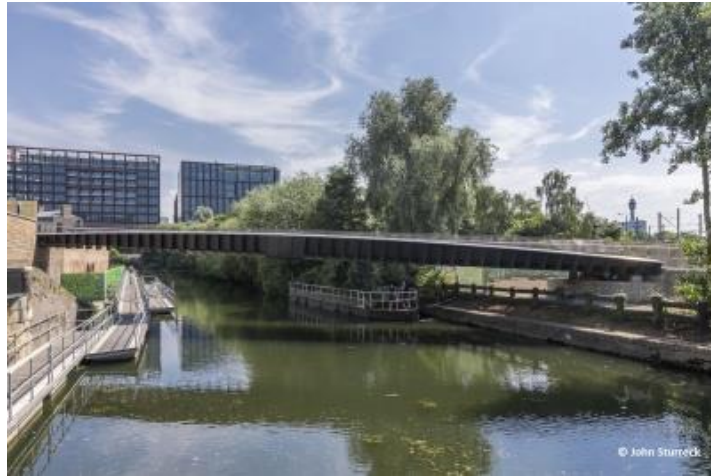
Figure 1-2 Somers Town Beam Bridge, London (SteelConstruction.info, n.d.)
