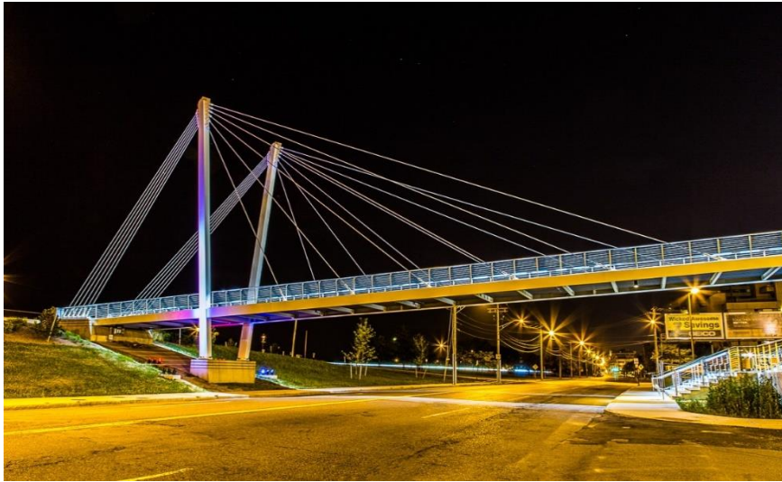
Figure 1-8 Christina and John Markey Memorial Pedestrian Bridge, Revere, Massachusetts (Duncan Galvanizing, 2018)
